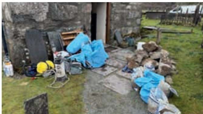
The builders yard outside the church
