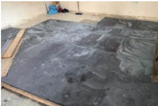
The Penrhyn Slate is laid
