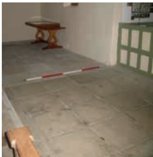
The concrete paving slab floor installed in 1963
