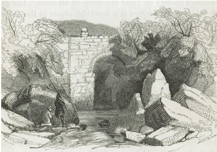
Hen Bont, which carried the new turnpike road over the Llugwy gorge near Gelli.
